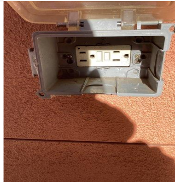
1 - Exterior Wall - GFCI/AFCI - Nov 13 2023 2:05PM - [REDACTED] CAPTION: Right outside community room
