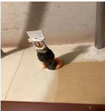
1 - Local Systems (Bldg) - Sprinkler Assembly - Nov 13 2023 1:16PM - [REDACTED] CAPTION: 3rd floor electrical room
